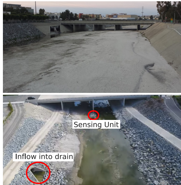
Fig. 6. Our testbed in Orange County, USA: a storm drain and the locations of sensing units.
